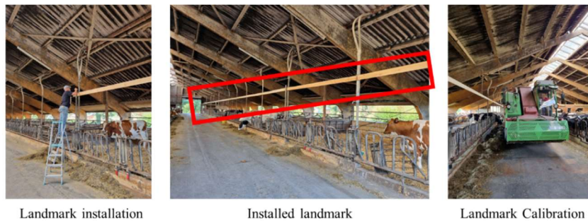
Fig. 2: Verti-Q system commissioning process
